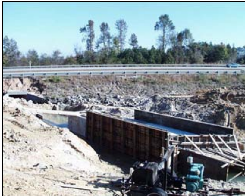
Figure 8. Culvert Construction
