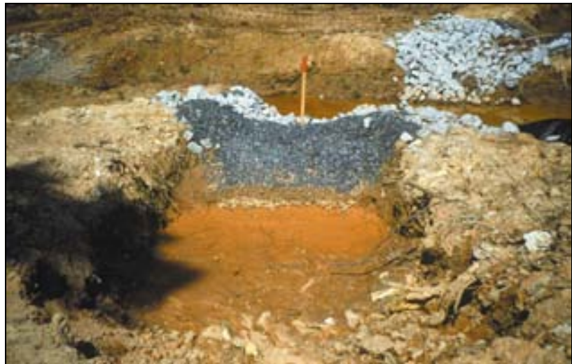
Figure 29. Temporary Rock Sediment Dam Type “B”
