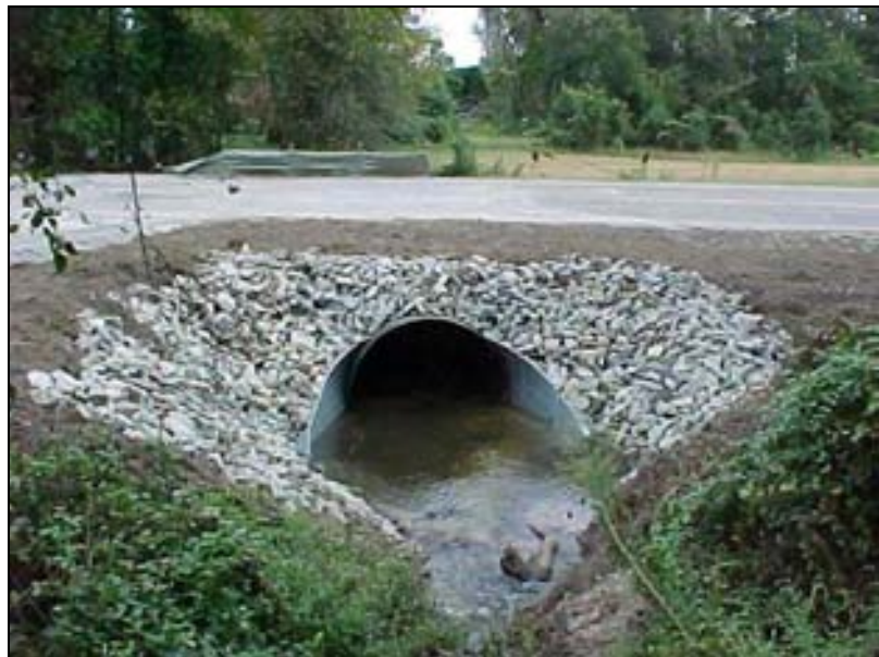
Figure 19. Completed Outlet Maintenance
