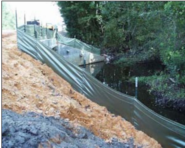
Figure 16. Headwall BMP Installation
