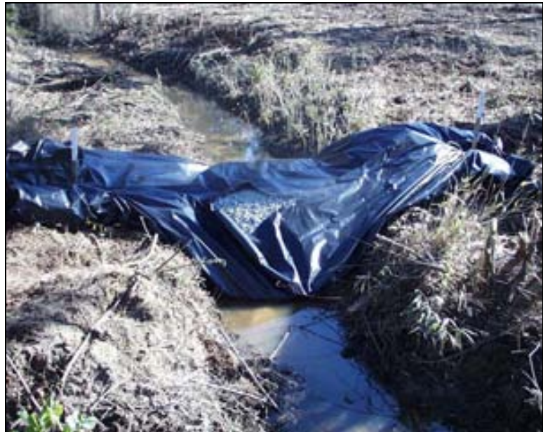
Figure 34. Installation of Stone with Impervious Fabric
