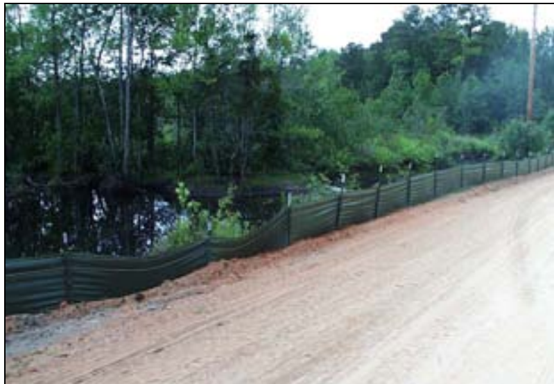
Figure 1. Typical Perimeter Erosion Controls
