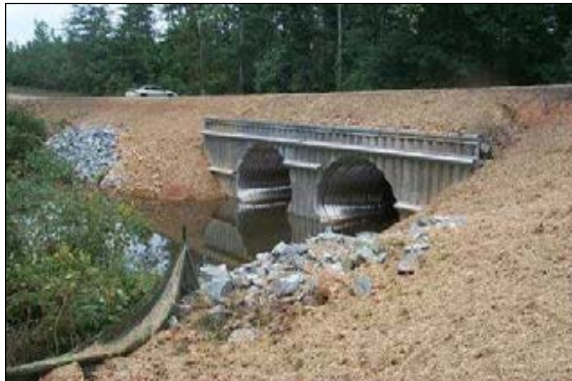
Figure 18. Completed Headwall Installation
