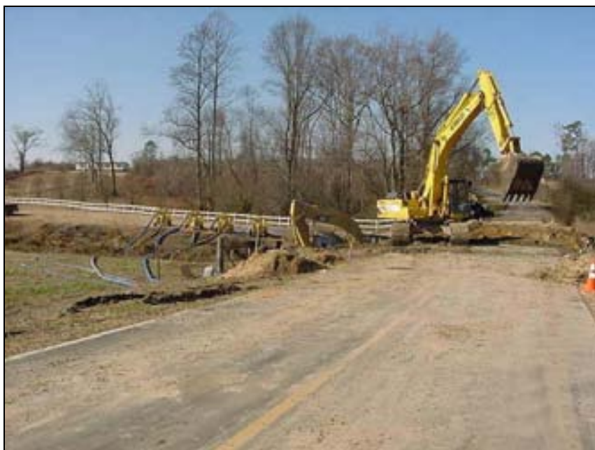
Figure 30. Bypass Pumping
