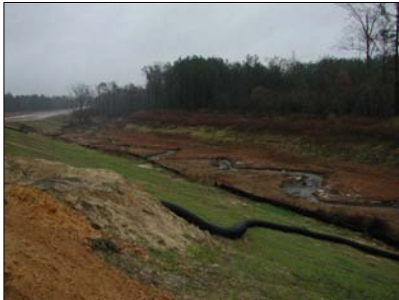
Figure 24. Completed Stream Channel Relocation
