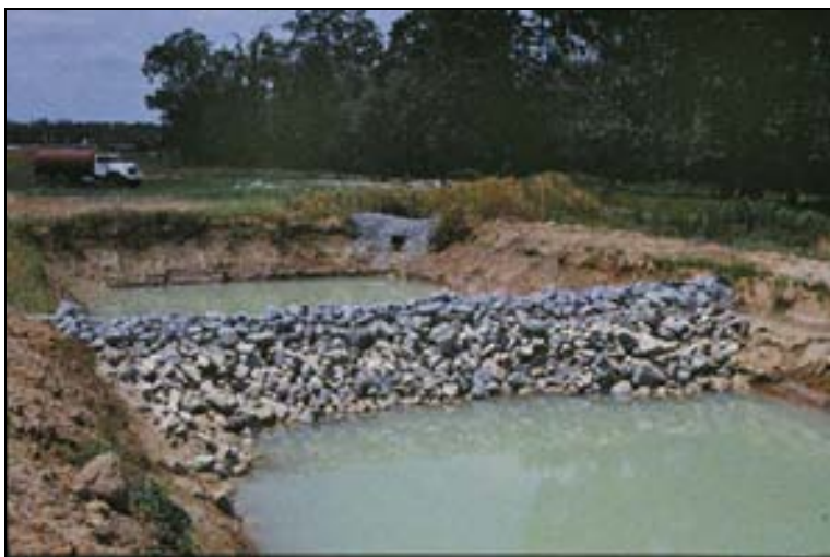
Figure 38. Stilling Basin for Pumped Effluent
