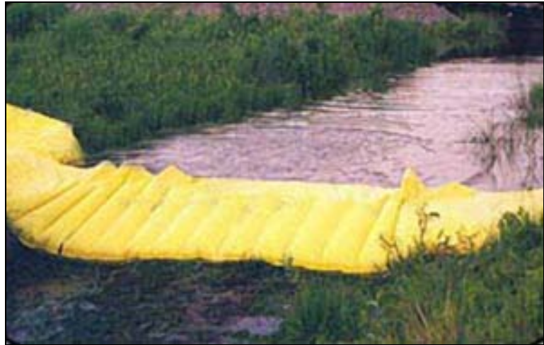
Figure 36. Prefabricated Dam
