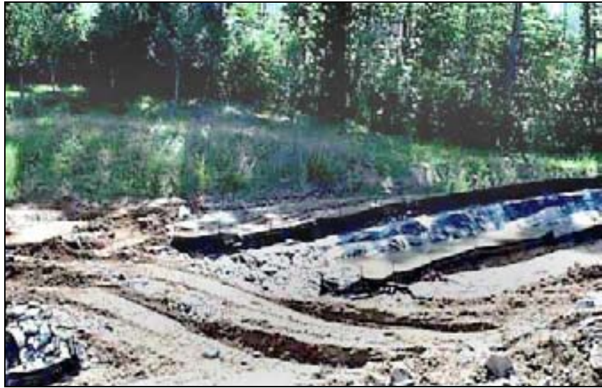
Figure 41. Temporary Piped Crossing
