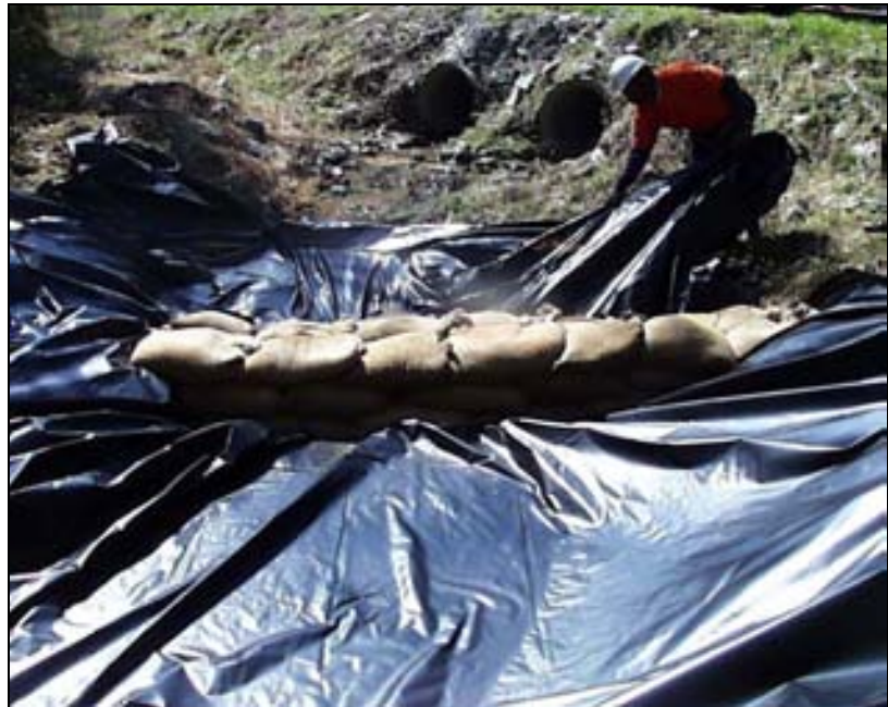
Figure 35. Sand Bag Installation
