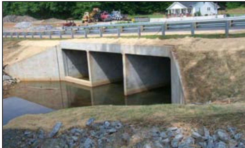
Figure 9. Completed Culvert Extension
