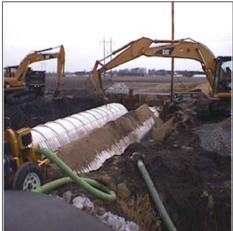
Figure 12. Pipe/Culvert Installation
