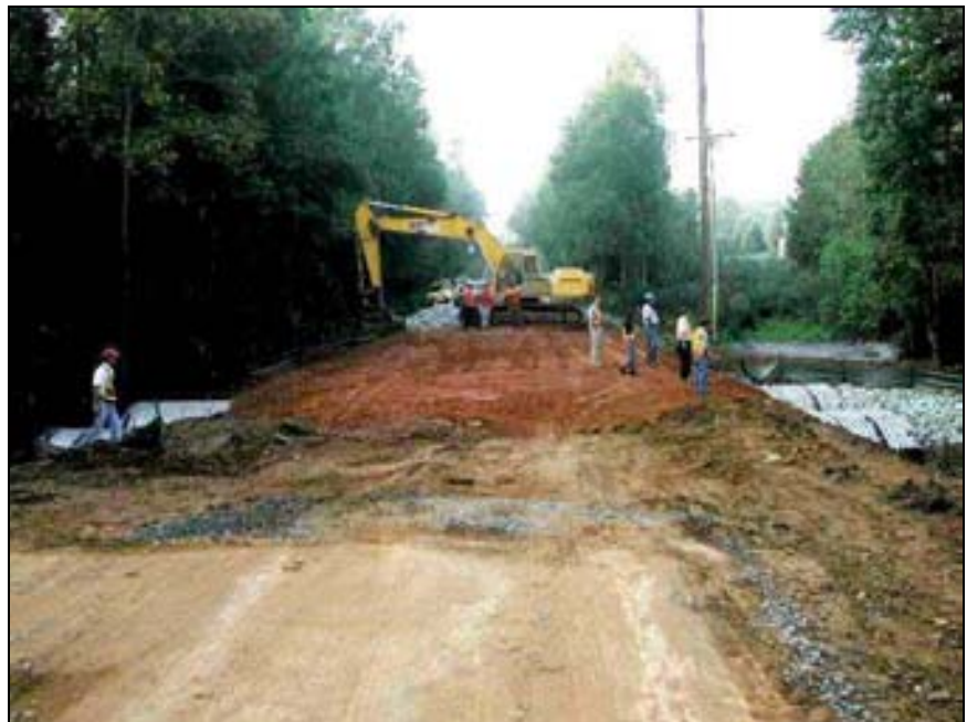
Figure 10. Pipe Repair/Replacement
