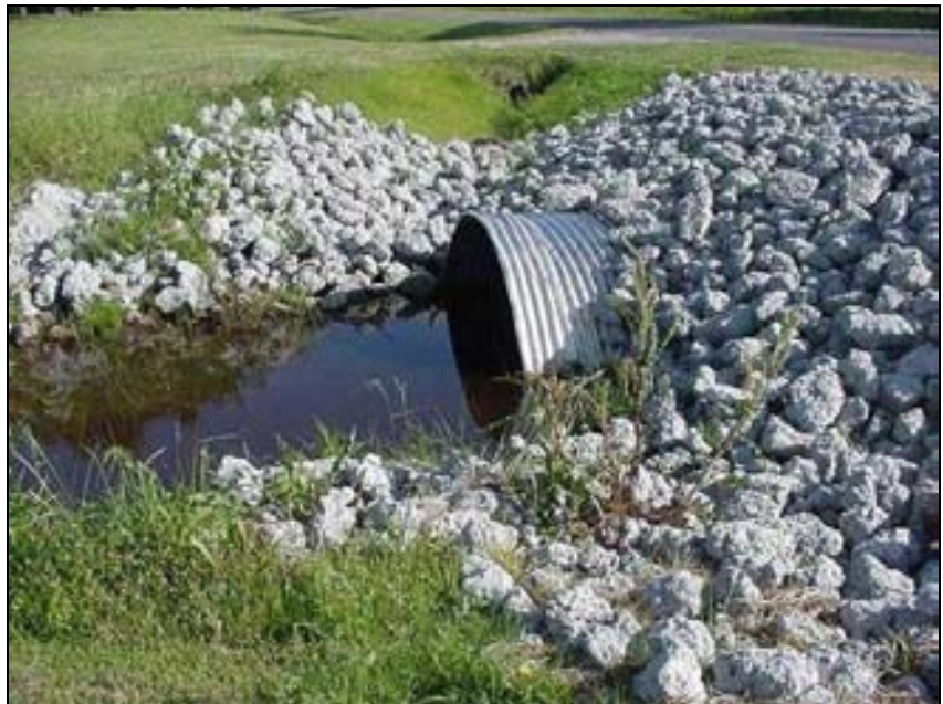
Figure 13. Pipe/Culvert Outlet Protection
