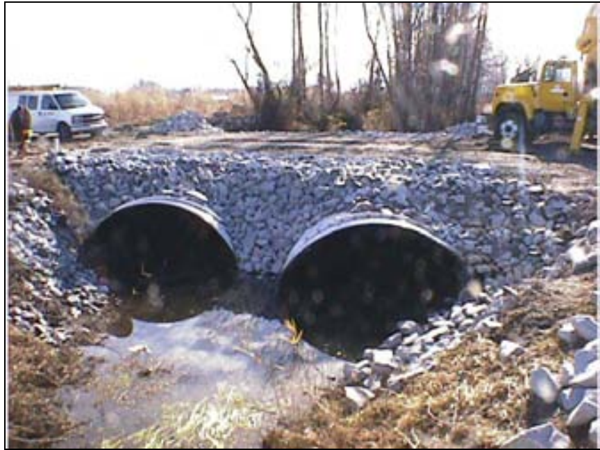
Figure 46. Riprap Slope Protection
