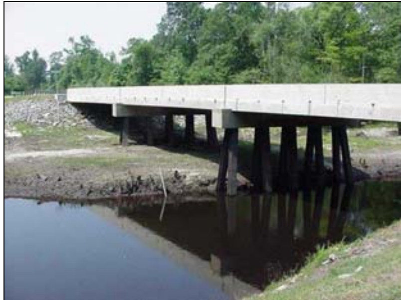
Figure 22. Completed Bridge Construction
