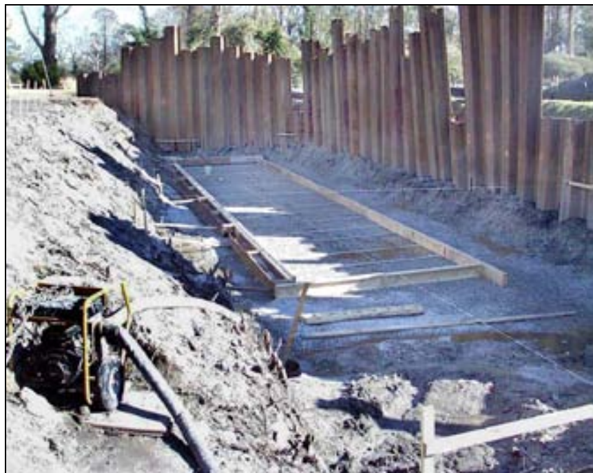
Figure 11. Pipe/Culvert Foundation Installation
