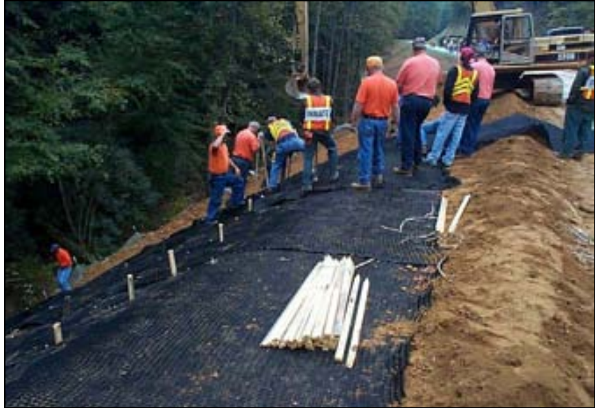
Figure 45. Erosion Control Blankets
