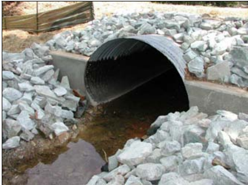
Figure 47. Riprap Outlet Protection
