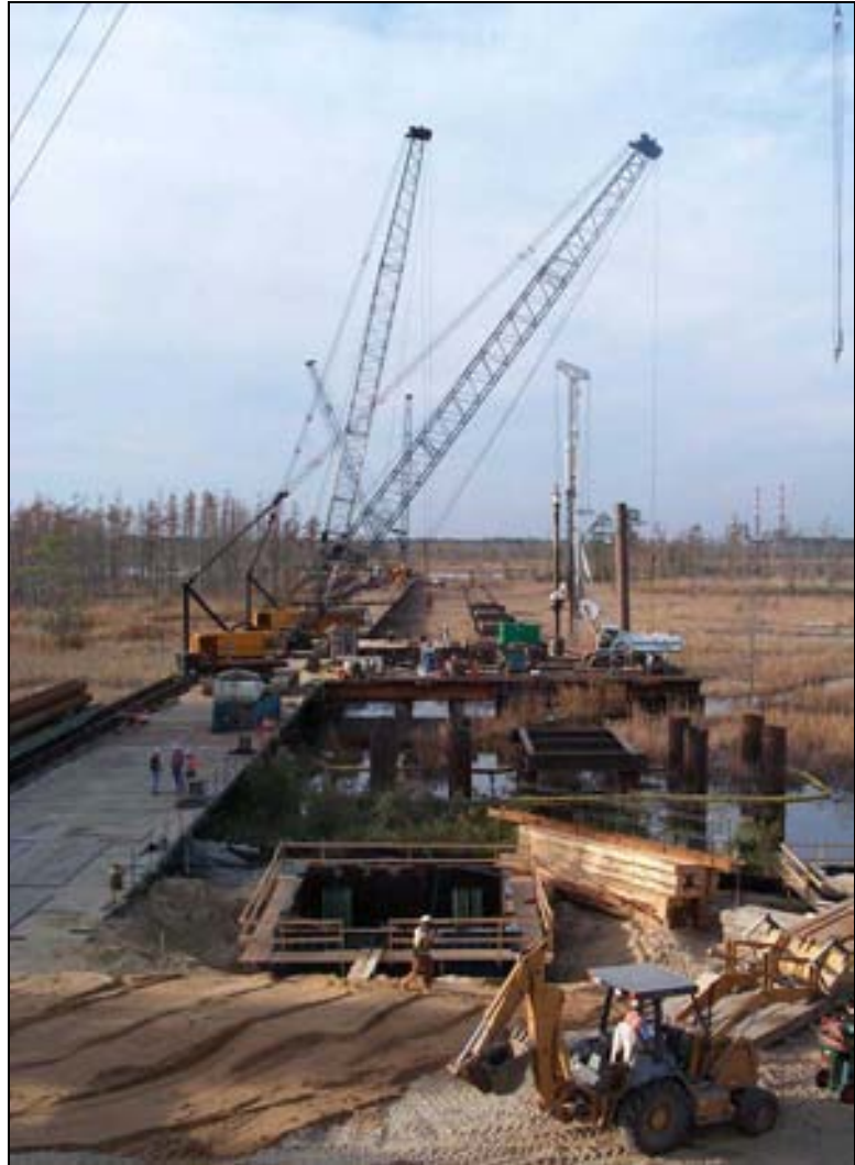
Figure 42. Temporary Access Bridge
