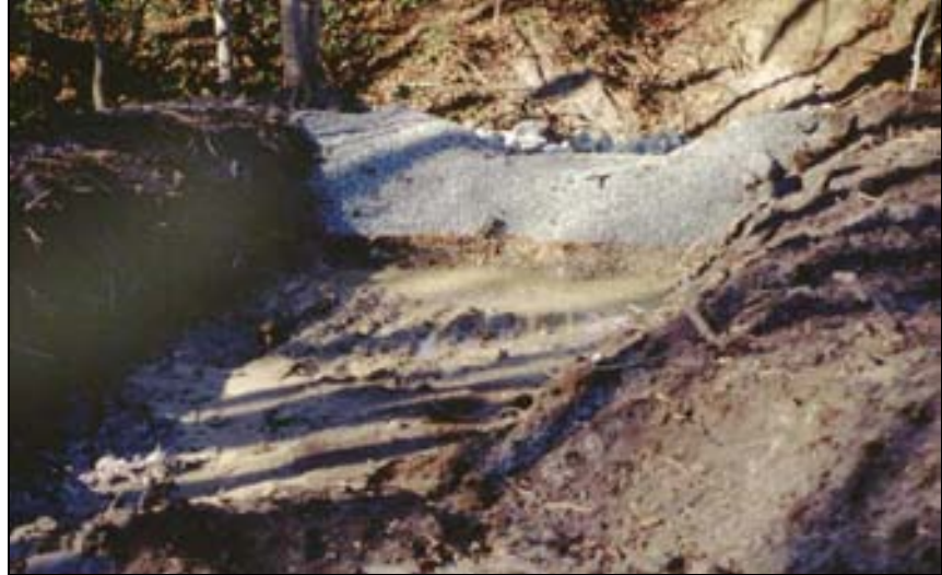
Figure 28. Rock Silt Check Type “A”
