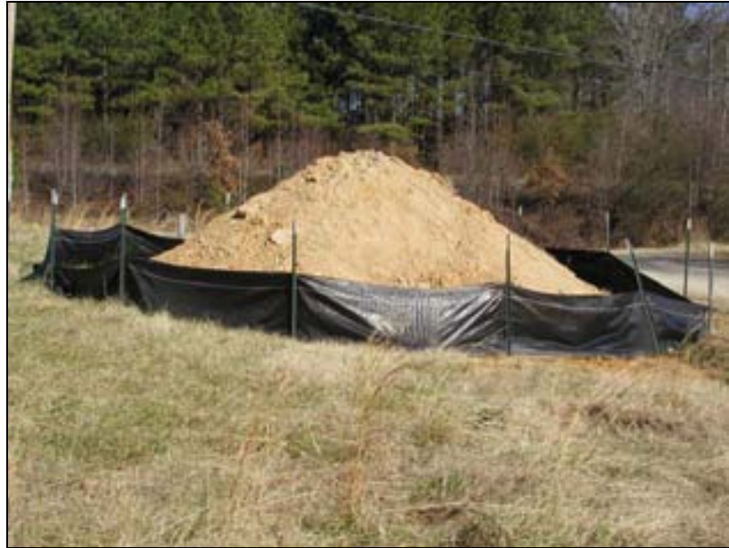
Figure 5. Typical Spoil Management
