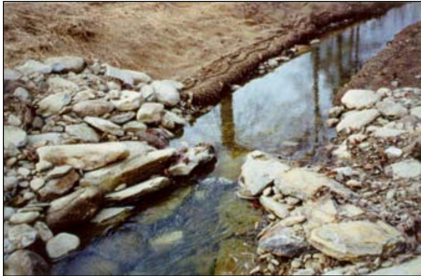
Figure 49. Cross Vane Rock Weir (looking upstream)
