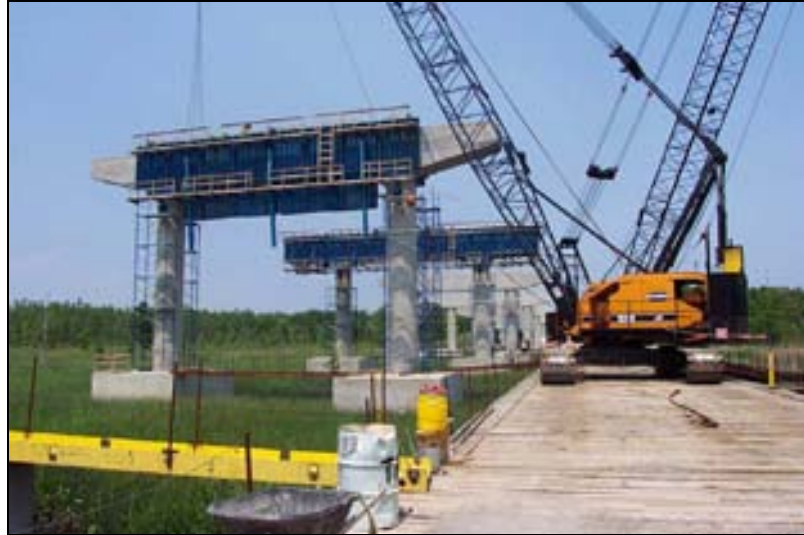
Figure 21 – Bridge Construction within Wetlands
