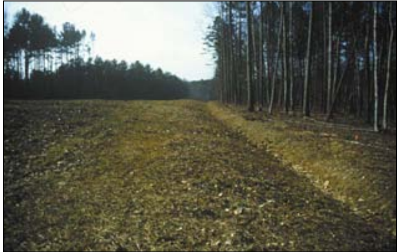
Figure 27. Temporary Silt Ditch
