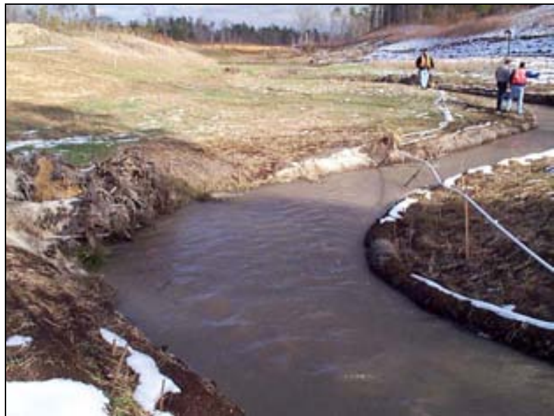
Figure 23. Stream Channel Relocation
