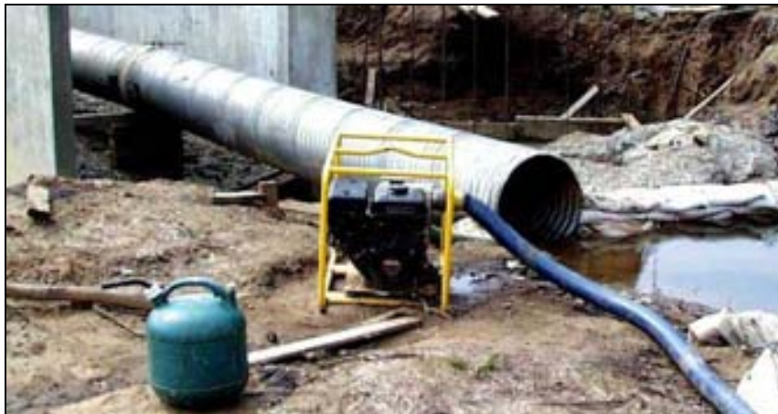
Figure 31 Suspended Bypass Pipe
