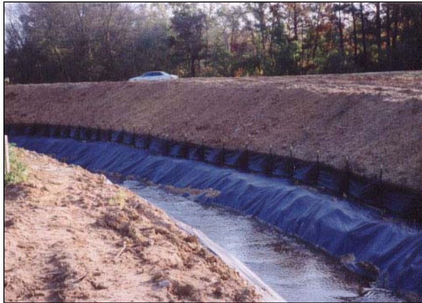
Figure 32. Fabric Lined Diversion Channel
