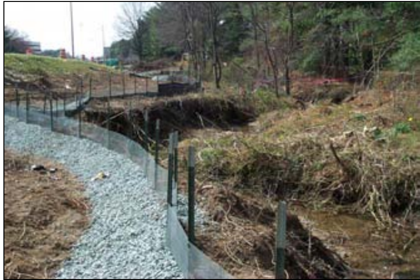
Figure 26 – Typical Special Sediment Control Fence
