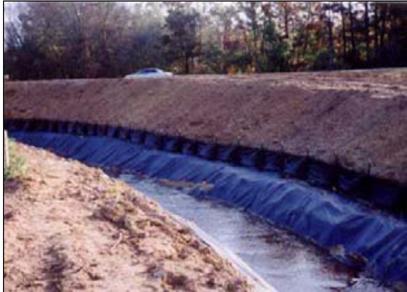
Figure 2. Water Course Diversion
