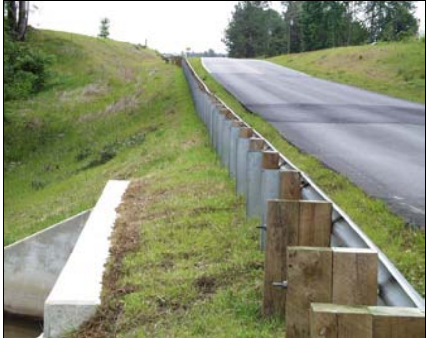
Figure 14. Completed Pipe/Culvert Installation
